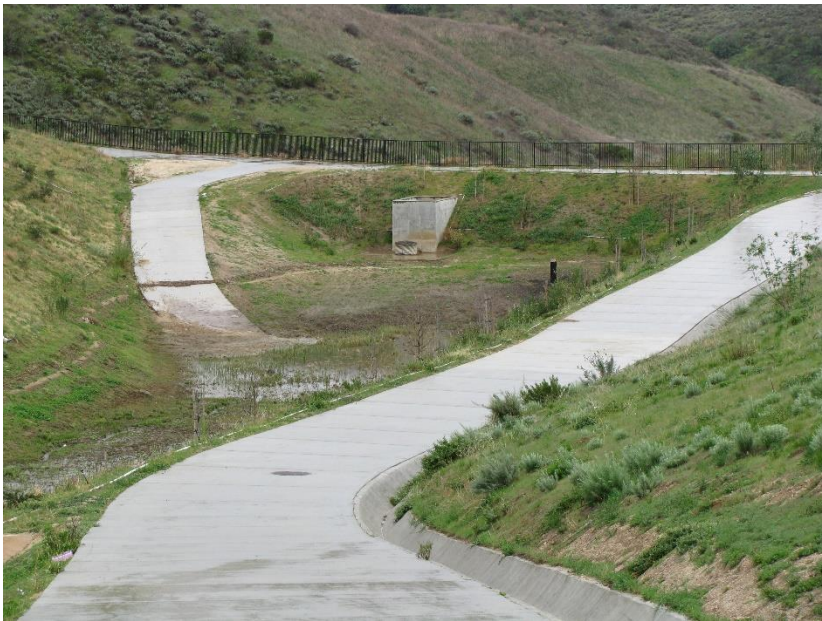
Figure 11: Extended Detention Basin
